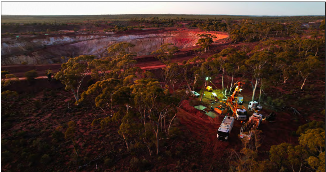
Figure 17. Geotechnical Diamond Drilling at Orion 1 (Looking East)
