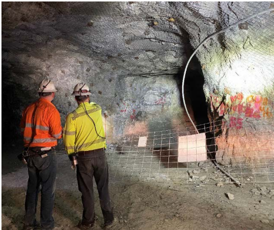
Photo 3 – Underground development drive showing good ground conditions
