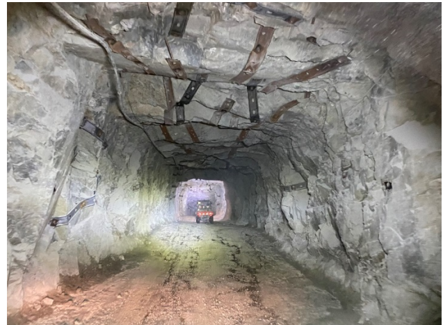
Photo 4 – Underground intersection showing good ground conditions, and existing services
