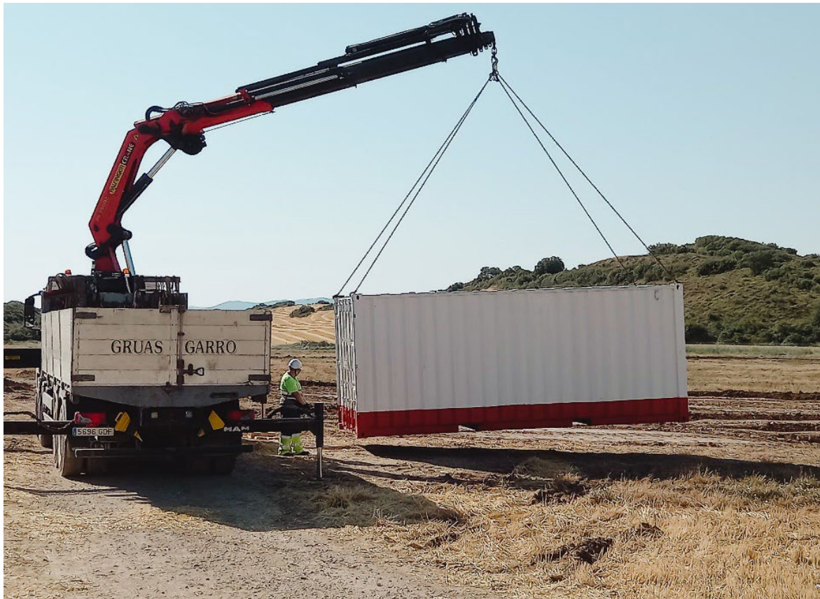
FIGURE 7: INSTALLATION OF THE ABOVE GROUND CONSTRUCTION STAFF FACILITIES AT MUGA MINE
