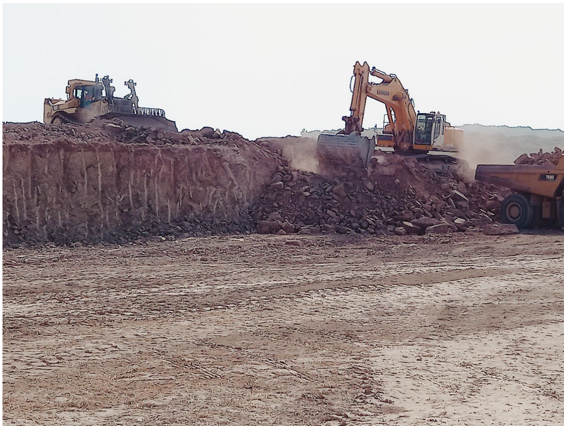
FIGURE 9: EXCAVATION OF THE MINE ENTRANCE
