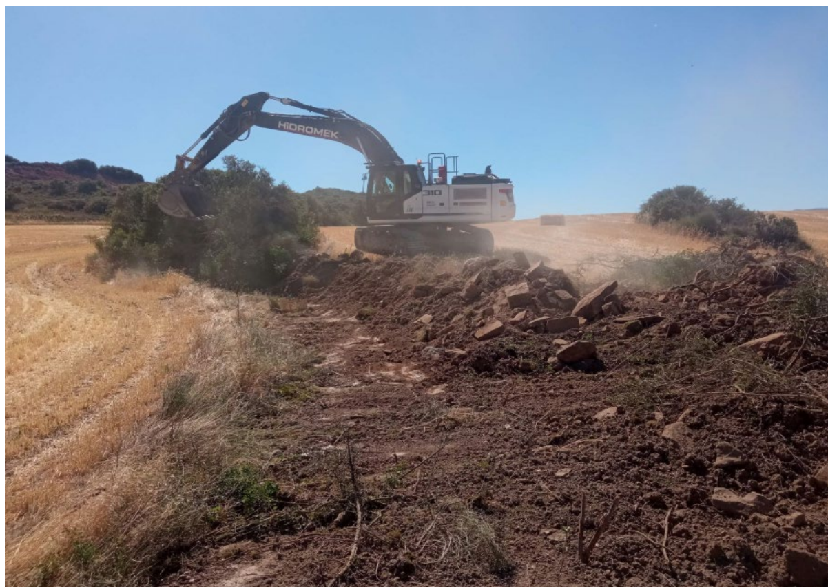
FIGURE 8: CLEARING AND STOCKPILING OF TOPSOIL AT MUGA MINE
