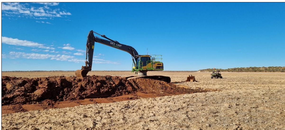
Figure 2: Establishing causeways for 2022 drilling campaign
