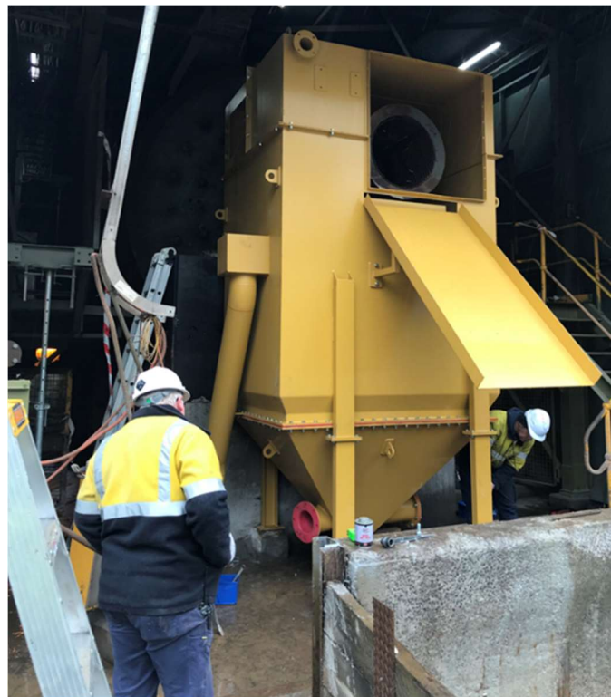
Figure 7: New discharge hopper installed in the SAG Mill building
