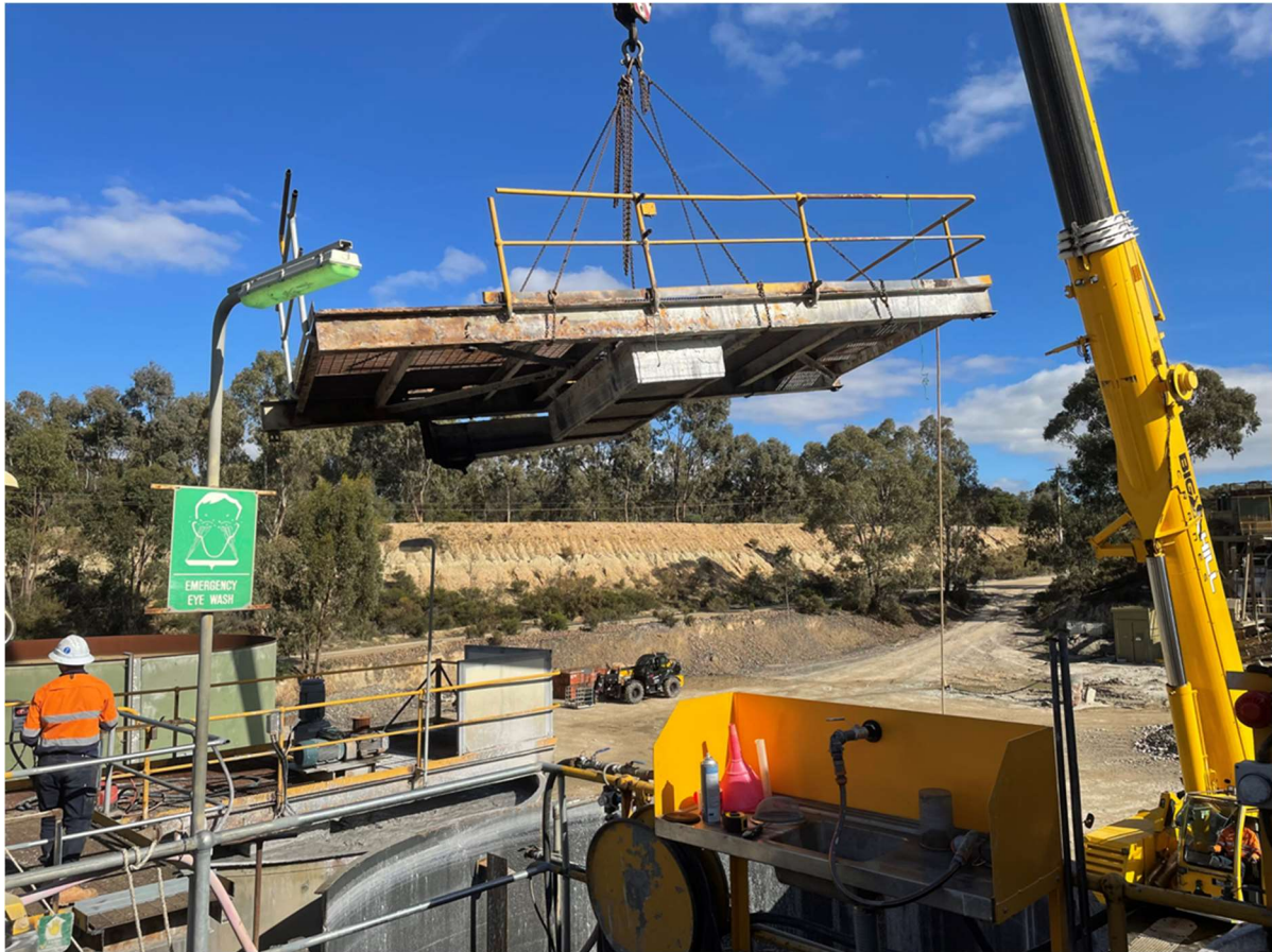
Figure 6: Old leach tank platform being removed
