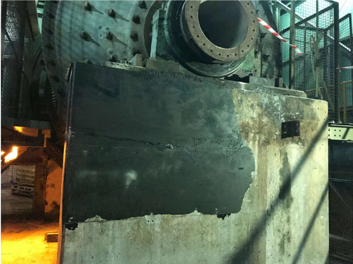
Figure 8: SAG Mill plinth/foundation repairs
