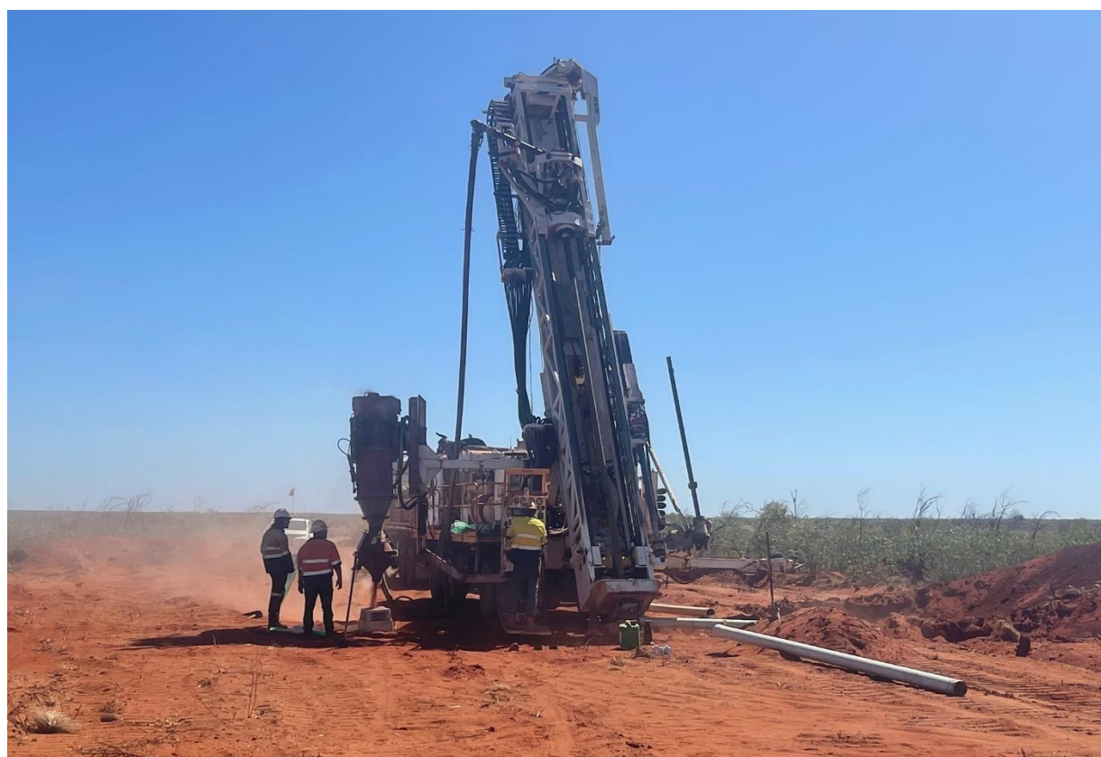
Figure 1 Impact Drilling Rig 1 collaring into CPRC015. The first drill hole of the Phase 2 RC Drill Program.
