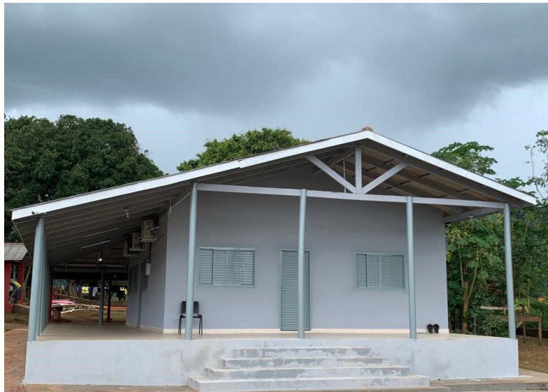
Figure 4 – New On-site Accommodation at Jaguar
