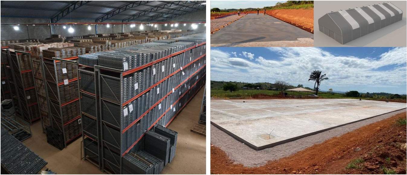
Figure 3 – Existing Core Shed (left) and build of new core shed (right)
