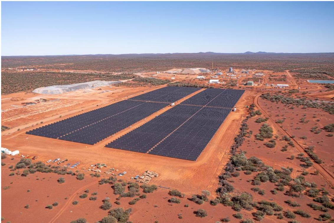
***Figure 9. 16,000 solar panels installed in solar farm.***
