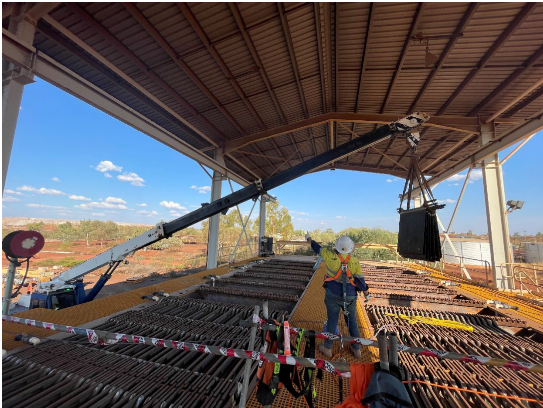
Image 7 / EW - Anode removal
