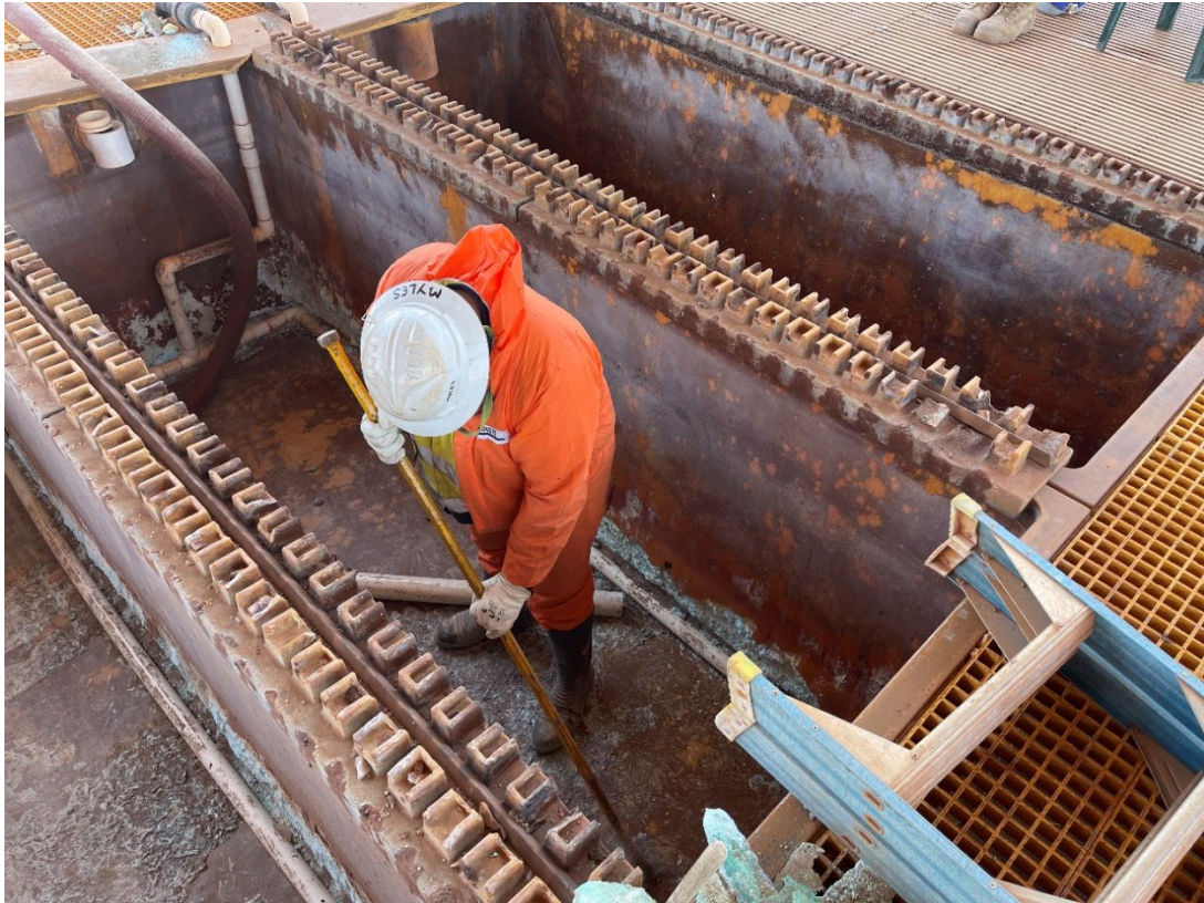
Image 8 / Cleaning out EW Cells post Hydro testing
