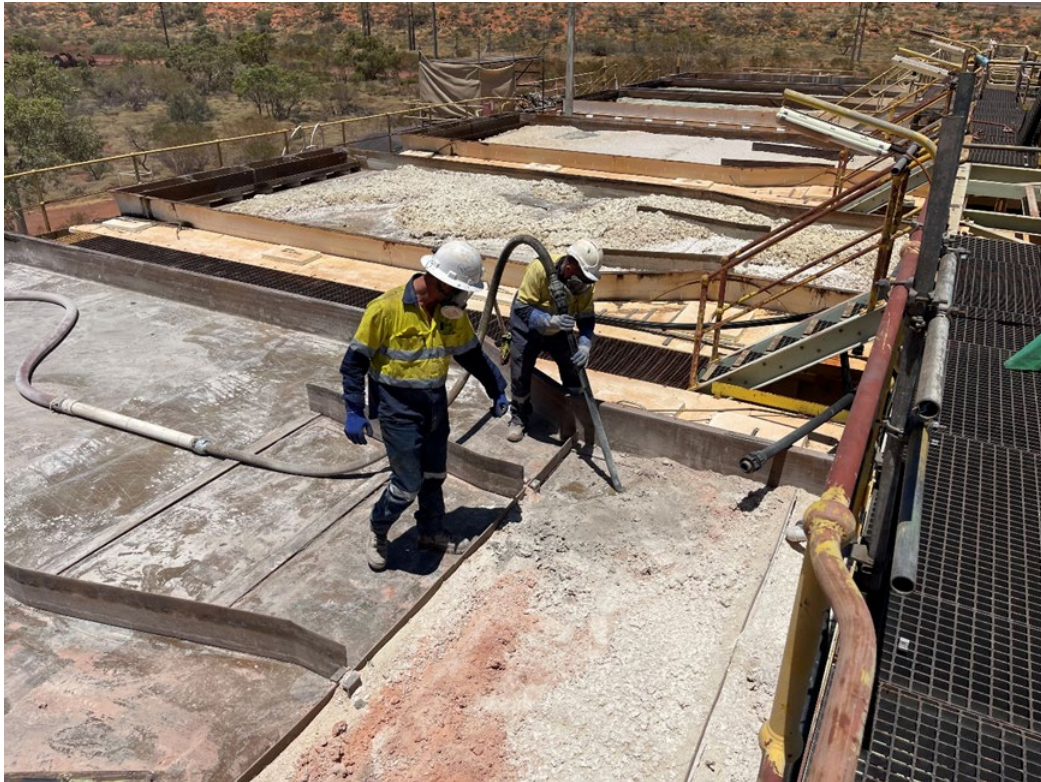
Image 2 / SX Mixer Settler clean-up top level
