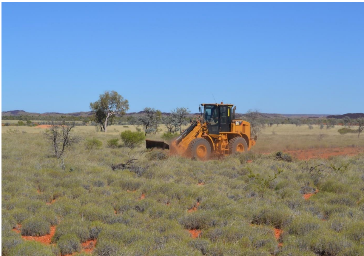
Photo 2 – Loader Clearing the Drill Lines at Shaw River
