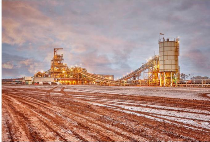
Figure 4: Mt Morgans Processing Plant
