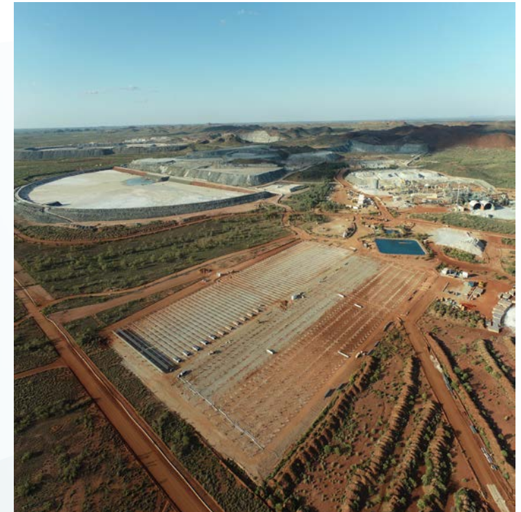
Pilgangoora Operation – Construction 6MW Solar Farm
