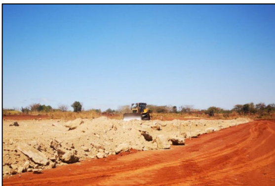
Figure 3: Construction of the TSF wall rockfill.
