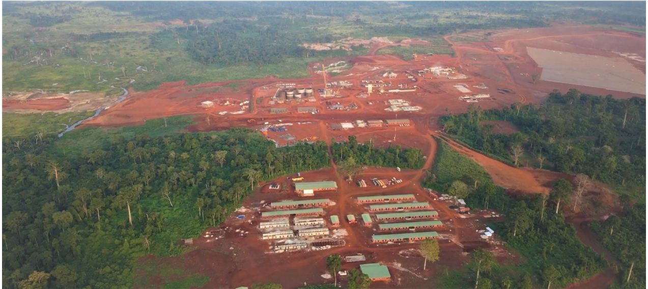
Figure 2: Overview showing construction status of Abujar Gold Mine 23 July 2022
