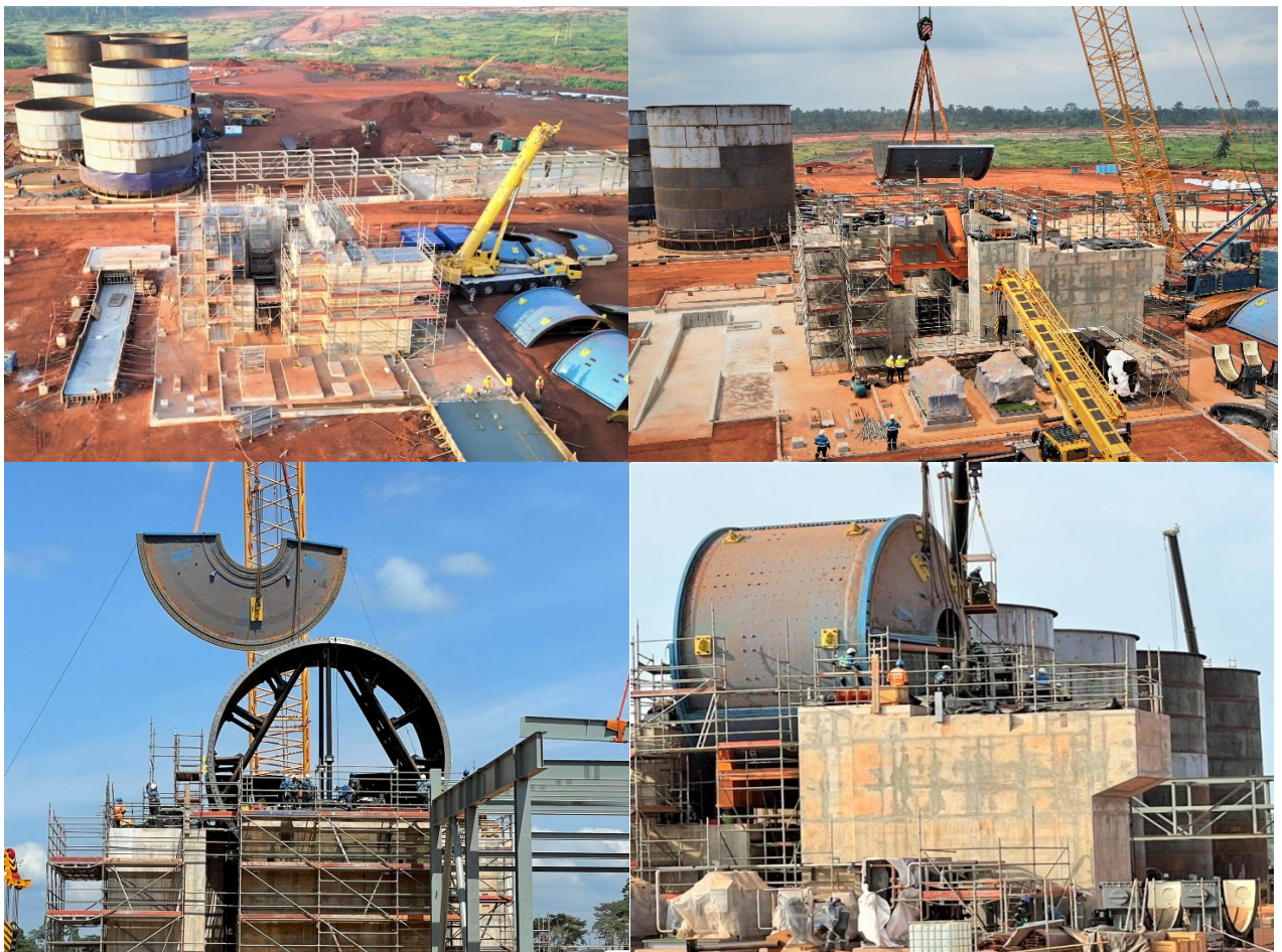
Figure 1: Overview showing construction activities on Abujar processing plant
