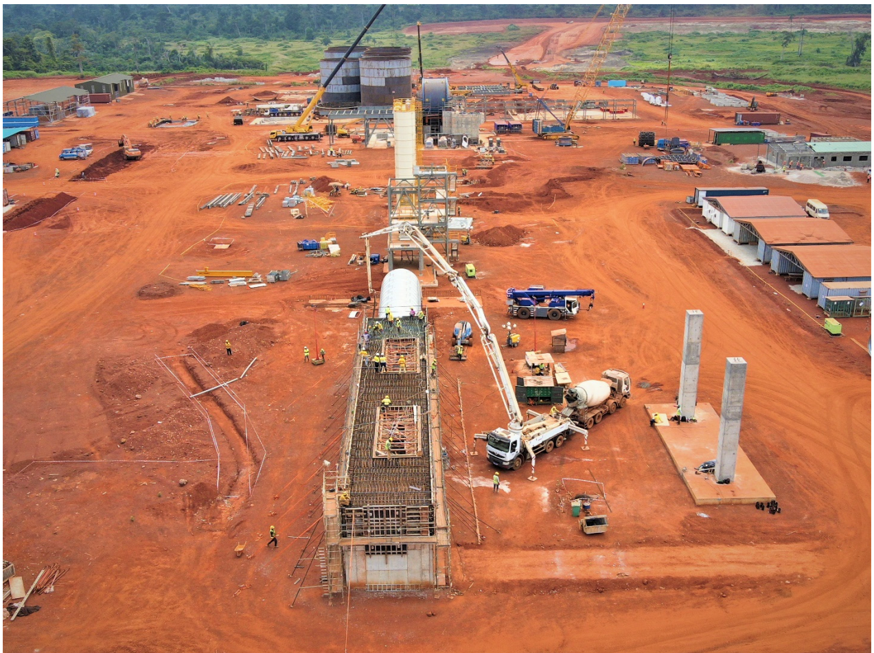
Figure 3: Main part of the Abujar Processing plant in construction 30 July 2022
