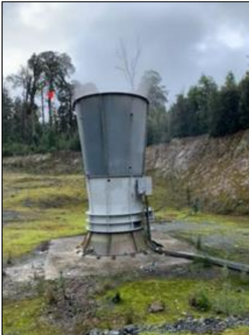
Figure 11: Vent fan #2 installation
