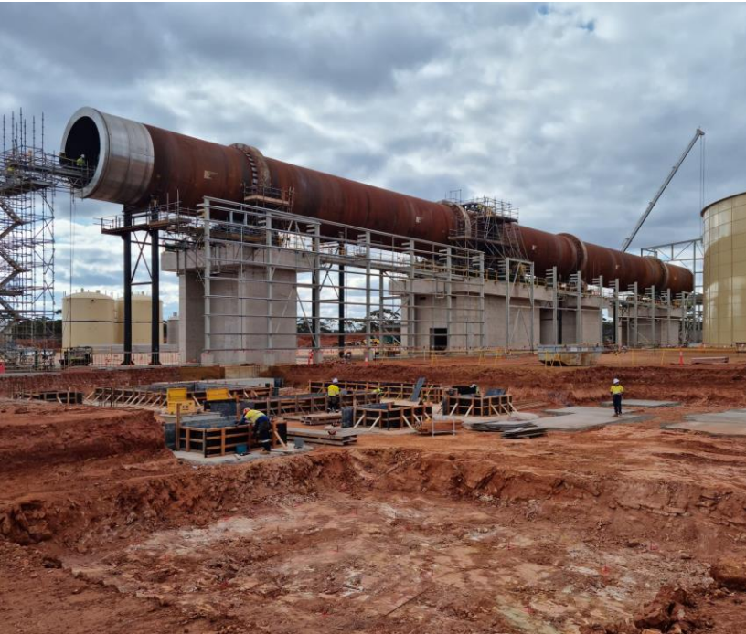
Kiln installed in position and has rotated under its own power
