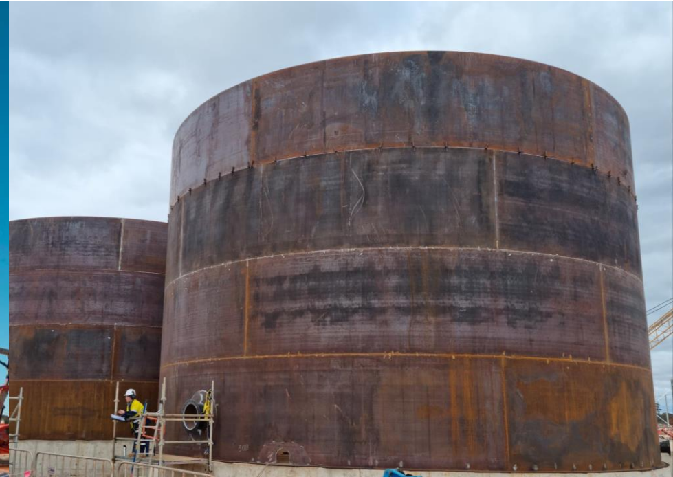
Fabrication of two 1300m 3 tanks complete
