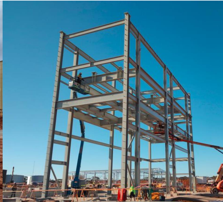
Filter building slab and foundations complete and structural steel progressing
