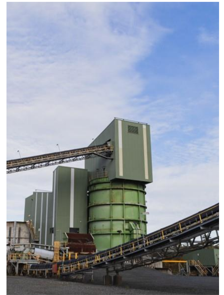
Crusher House and Fine Ore Bin
