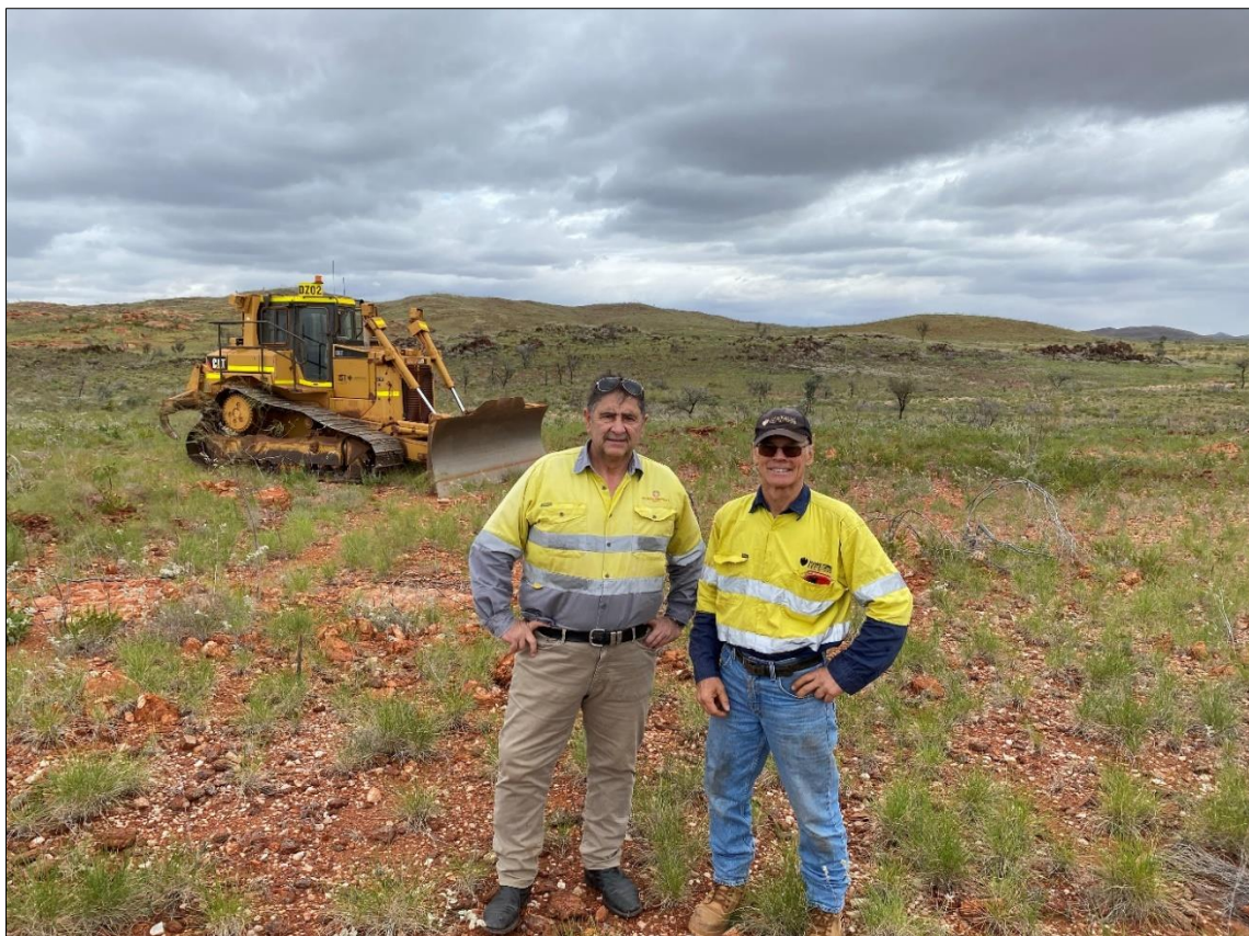
Photo 1 – George Karageorge (Managing Director left) and Grant Brooks (right, owner of Limestone Station) commencement of the drill pads preparation over the Sister Lithium Project
