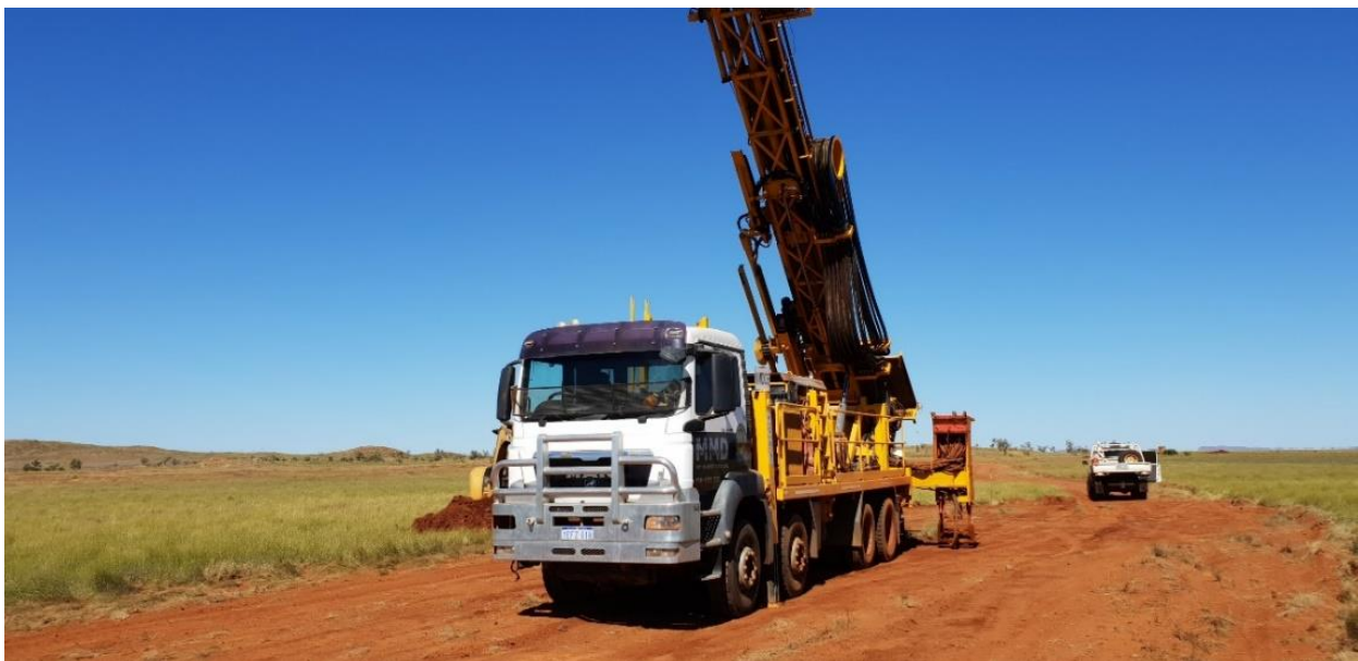
Diamond drilling rig on drill site 22SBDD001, looking south towards Sherlock Bay nickel sulphide resource
