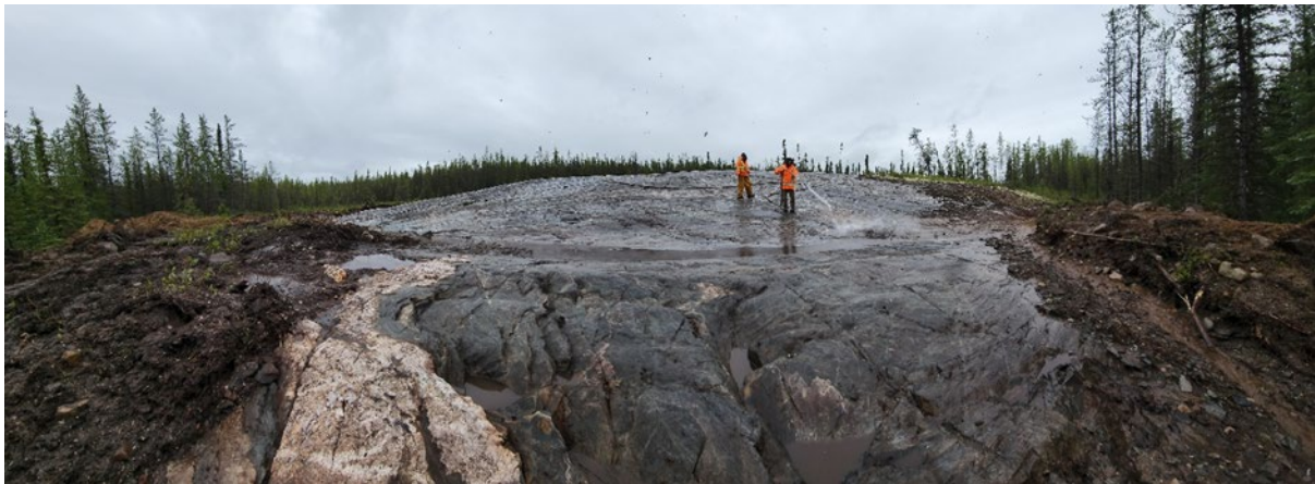
Figure 1 & 2 – preliminary stripping of vegetation to expose Cancet main dyke
