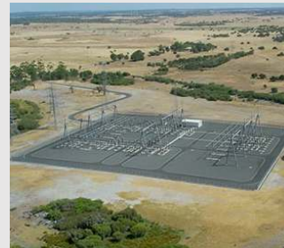
Landwehr Terminal SWIS 3.5km from BSS
