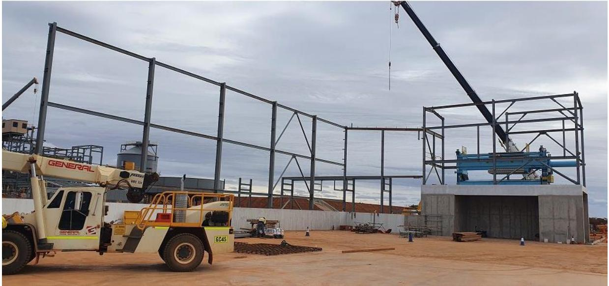
**Figure 11**– Concentrate filter and shed construction.
