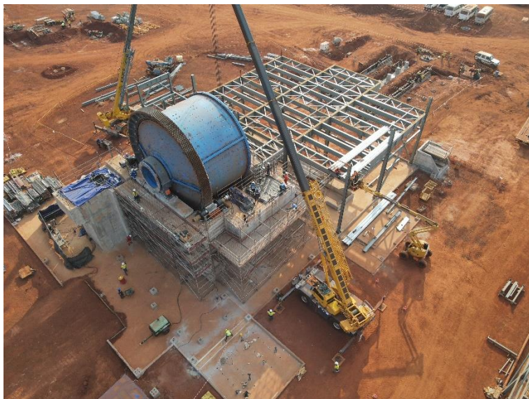
Figure 1: Overview showing construction status of Abujar's SAG mill and CIL tanks as at 13 August 2022
