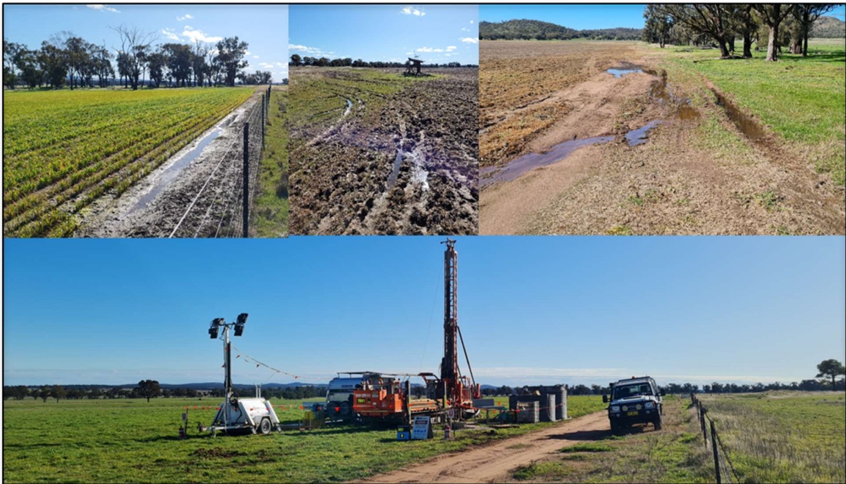
Figure 2: Access conditions (above) at Narraburra and Diamond drill rig on hole GNBDD001 (below).
