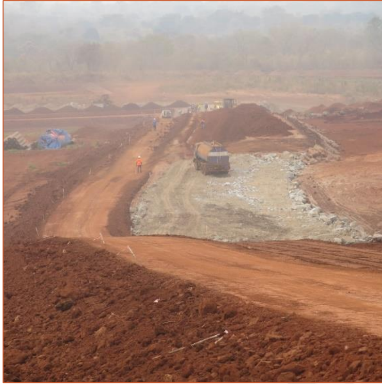
Figure 8: Construction of the tailings storage facility retainer walls.
