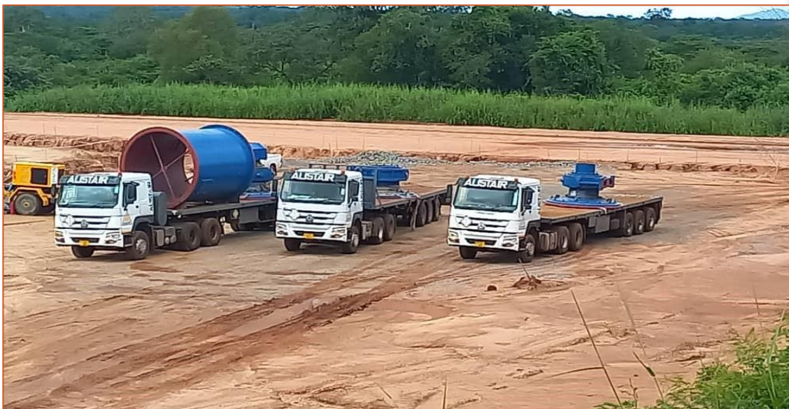
Figure 2: Rod mill arriving on site in April 2022.
