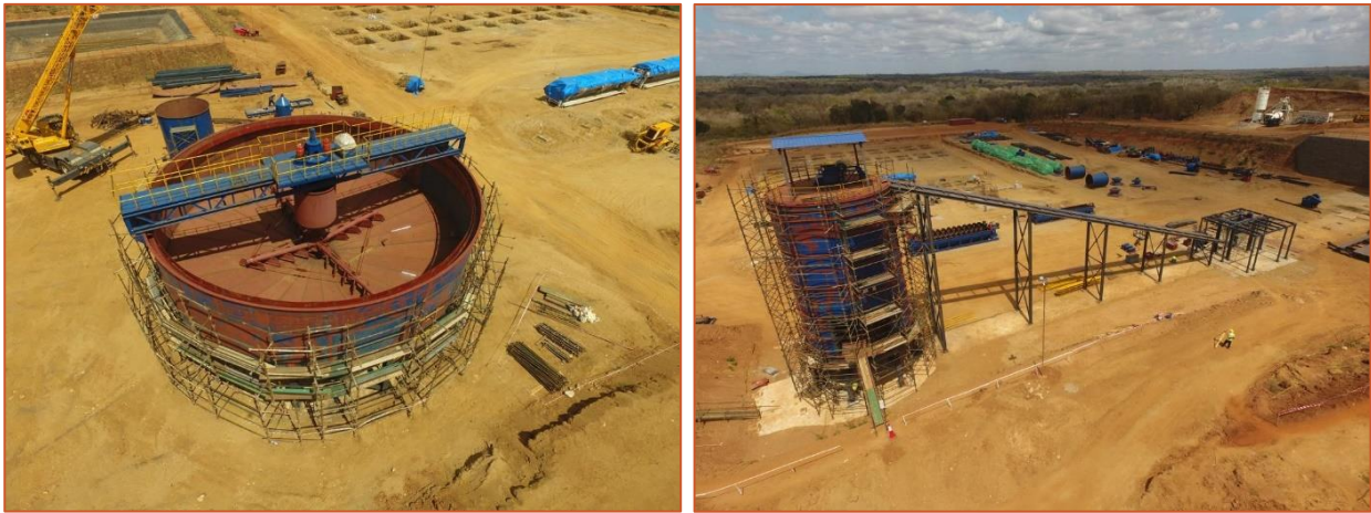
Figure 3: Thickener (left) and fine-ore bin with feed conveyor structure (right) .
