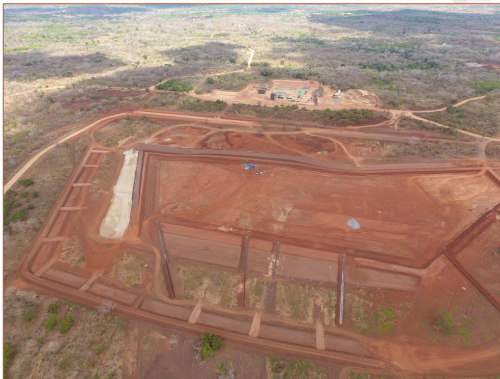
Figure 7: Oblique view from the north of the TSF area in mid-August. Processing plant in the background with starter pit visible on the top right of the photo.
