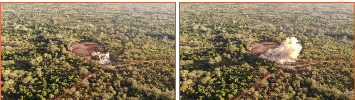
Figure 9: Blast sequence at the starter pit looking south. The main super high-grade zones are approximately 30m to 50m to the east (left) of the blast zone and strike NE-SW.
