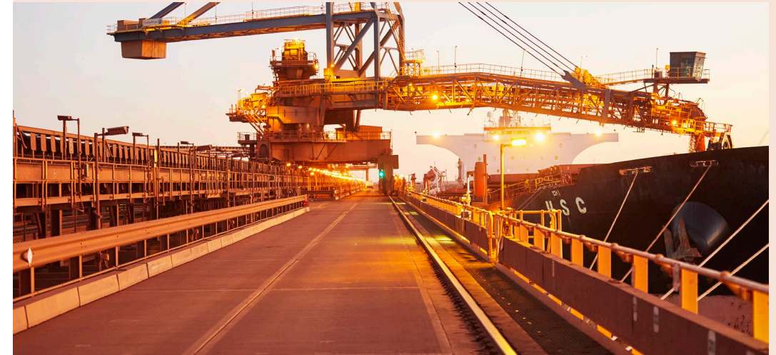
FMG Port Facilities, Pilbara region of WA
