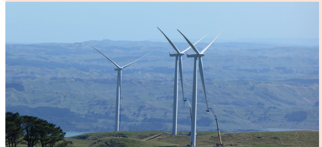
Meridian Energy's windfarm maintenance, New Zealand
