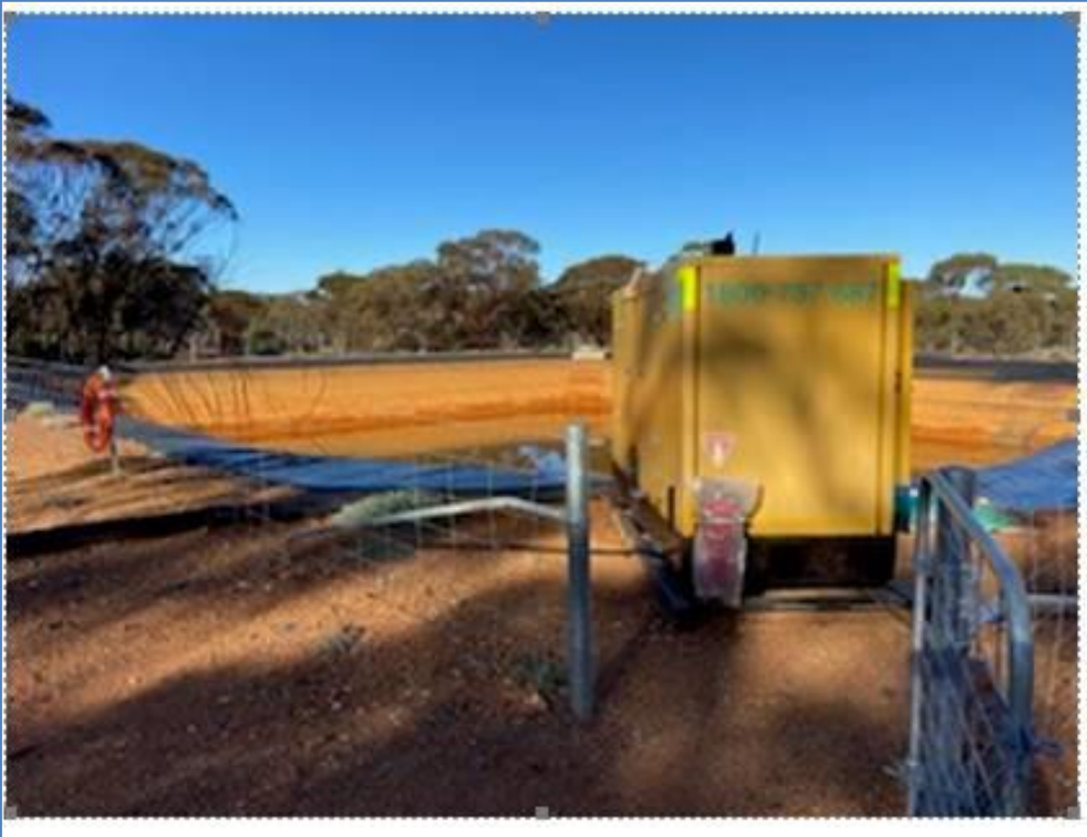
Figure 4: Turkey's nest located at the Andrew's Shaft providing readily available water source
