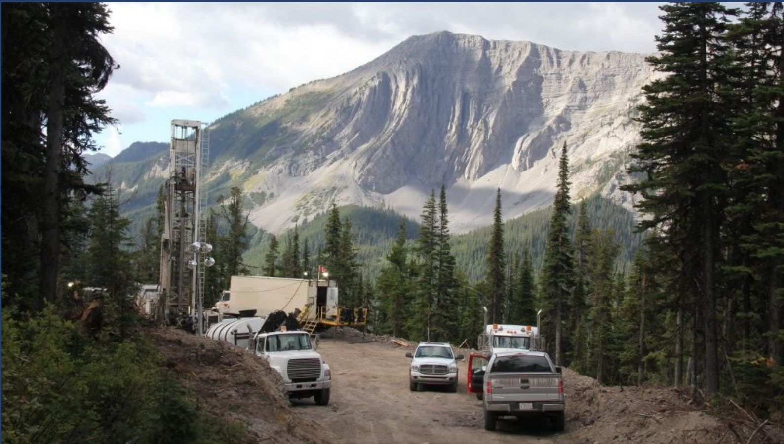
Crown Mountain – exploration drilling in North Pit
