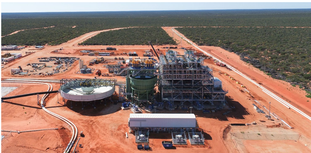
Figure 1 Construction verification and pre-commissioning of Coburn's Wet Concentration Plant progressing rapidly
