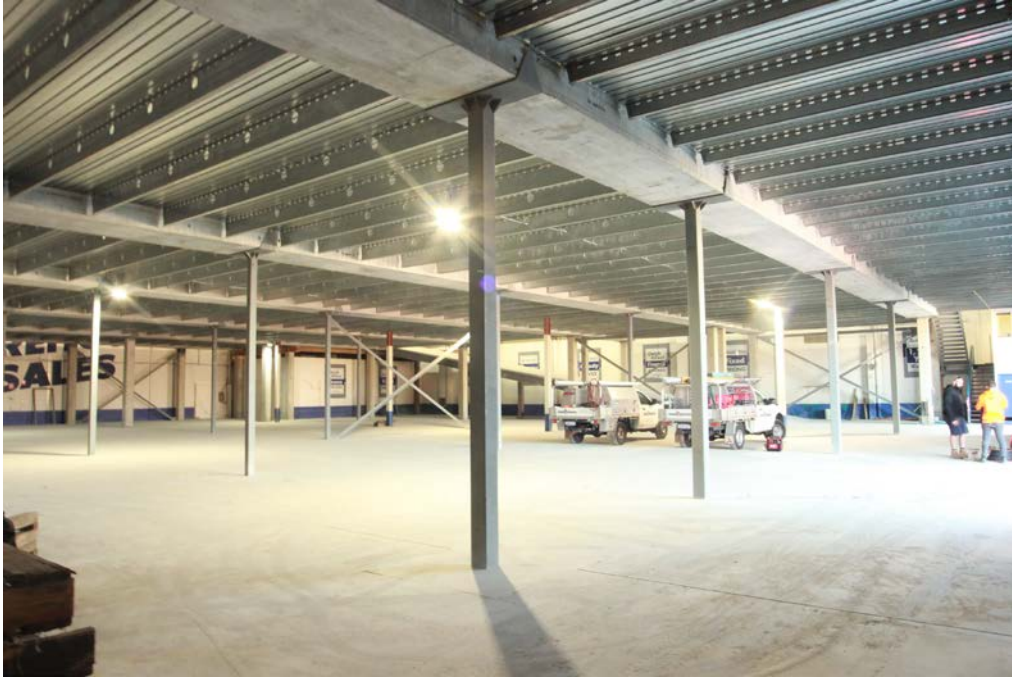
Picture 2. Underside of structure showing CVB and Slab System
