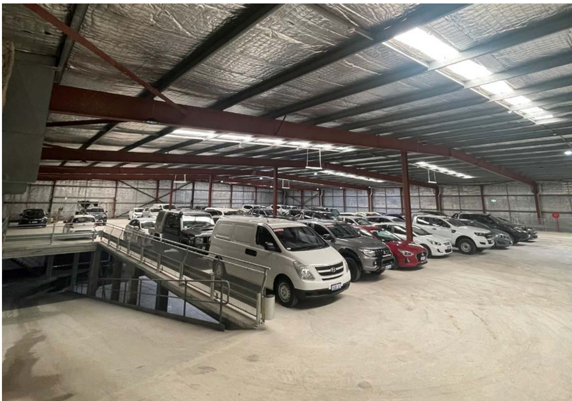
Picture 3. Completed mezzanine level in use
