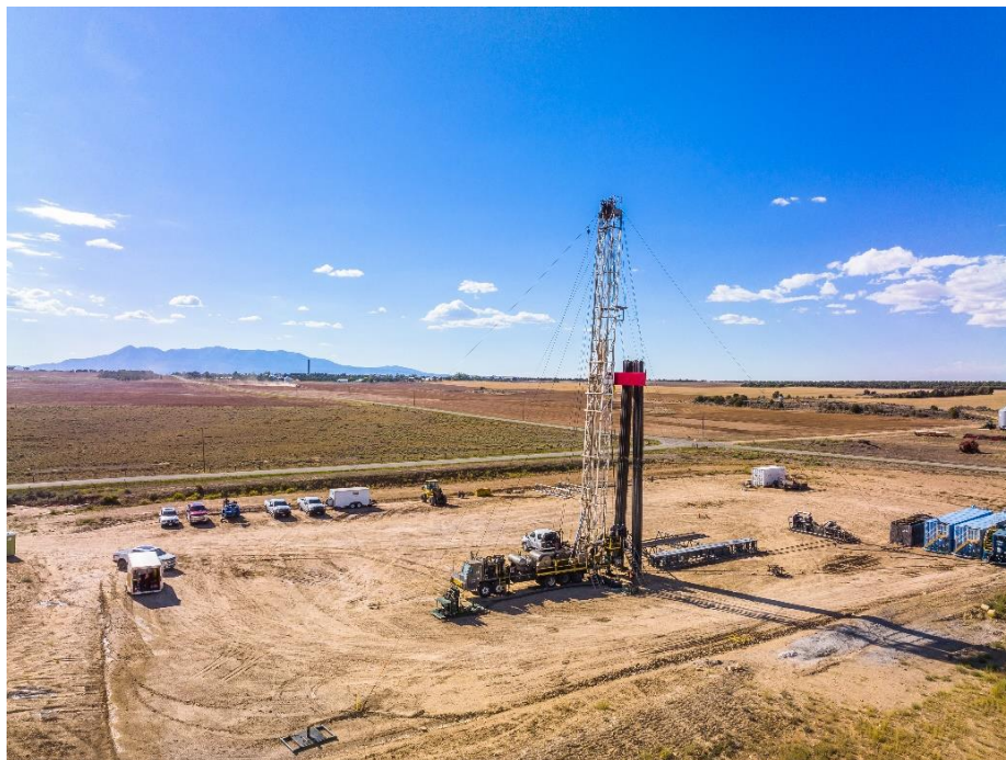
Work-over Rig on Jesse#1A with the Abajo mountains in the background
