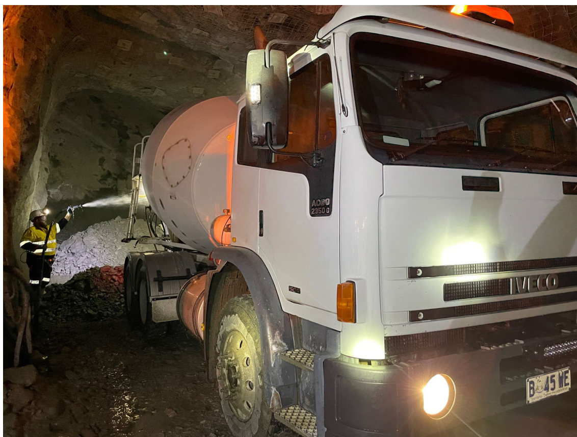
Figure 6. Cemented Rock Fill (CRF) operation at Avebury
