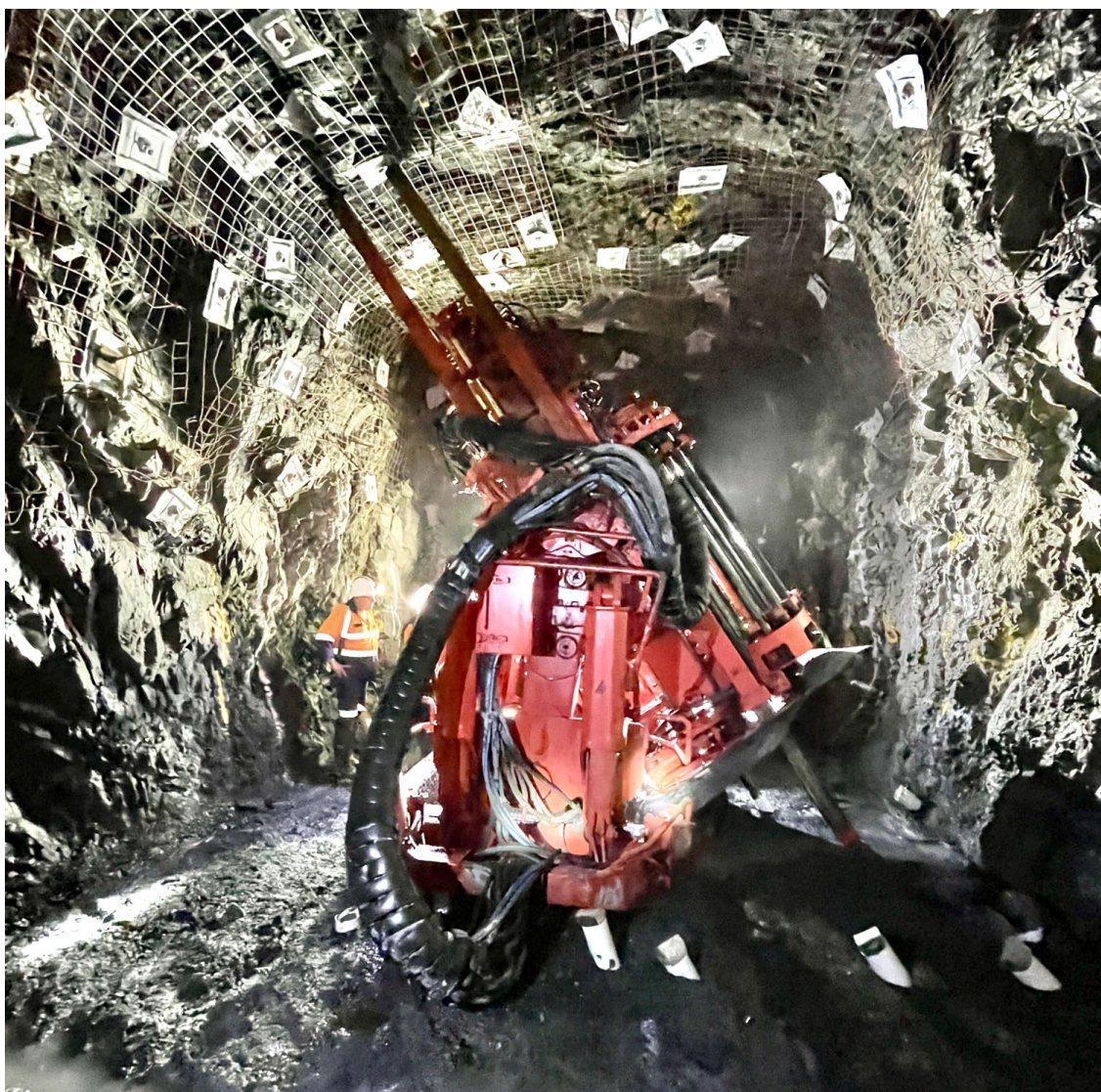
Figure 7: Longhole rig drilling stope production holes at Avebury
