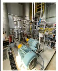
Inside the H2Sweet Plant at 2-29. This facility safely extracts the hydrogen sulphide ( $H_2S$ ) from the natural gas and converts it to a solid sulphur cake that can be disposed of safely (or potentially sold with additional processing). This process is one of a kind and reduces operating costs by \$1.30/mcf compared to triazine operations and significantly reduces the comparative environmental impact of triazine disposal.
