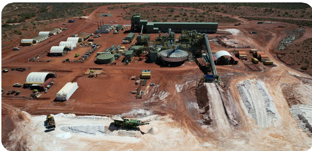
SOP Purification Plant ready for restart, with newly installed mobile crusher on the ROM pad in the foreground
