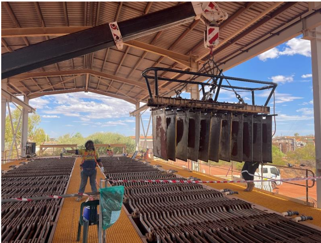
Image 2 / EW - Removal of Cathodes
