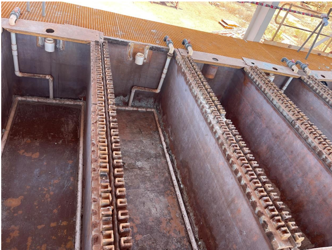
Image 4 / Cleaned EW Cells ready for condition inspection
