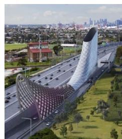
Westgate Tunnel Switchboards – Trivantage Manufacturing Over $10m
