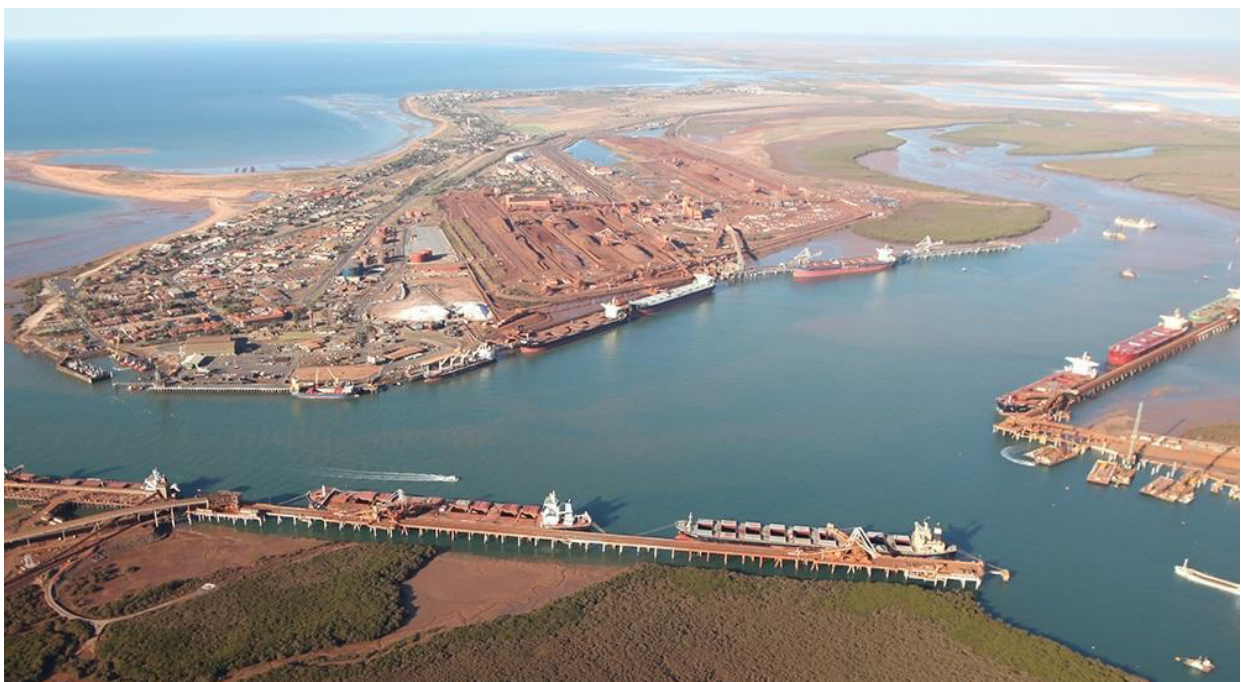
Image: Port Hedland Iron Ore Export Facilities
