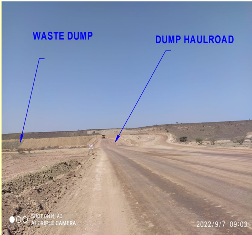
Haul road (30m width) leading to gossan dump
