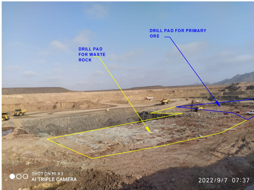
Waste rock and ore drill pad at 440 mRL
