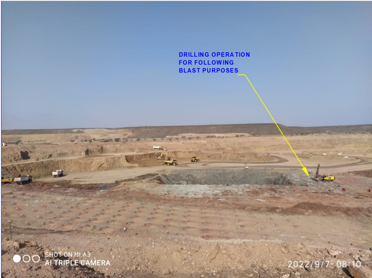
Drilling machine in operation
