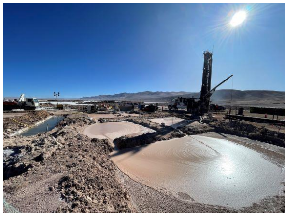
Figures 1-2. Rincon Lithium Project – Production Well Rotary Drilling Works
