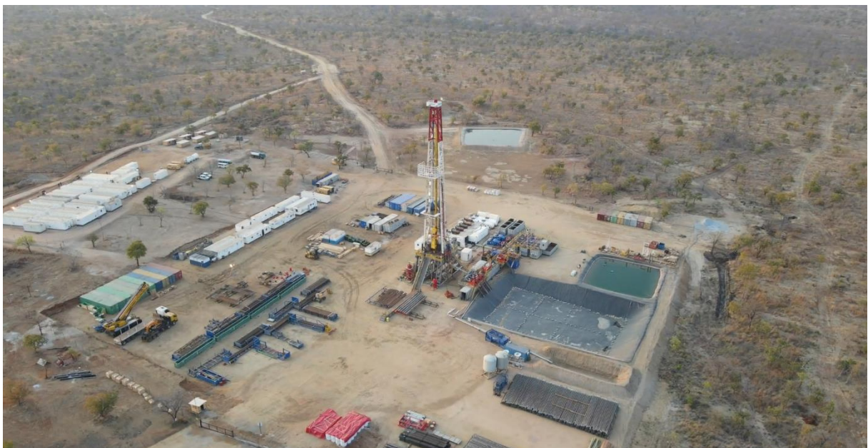
Figure 2 - Exalo Rig 202 at Mukuyu-1 wellsite preparing to commence drilling
