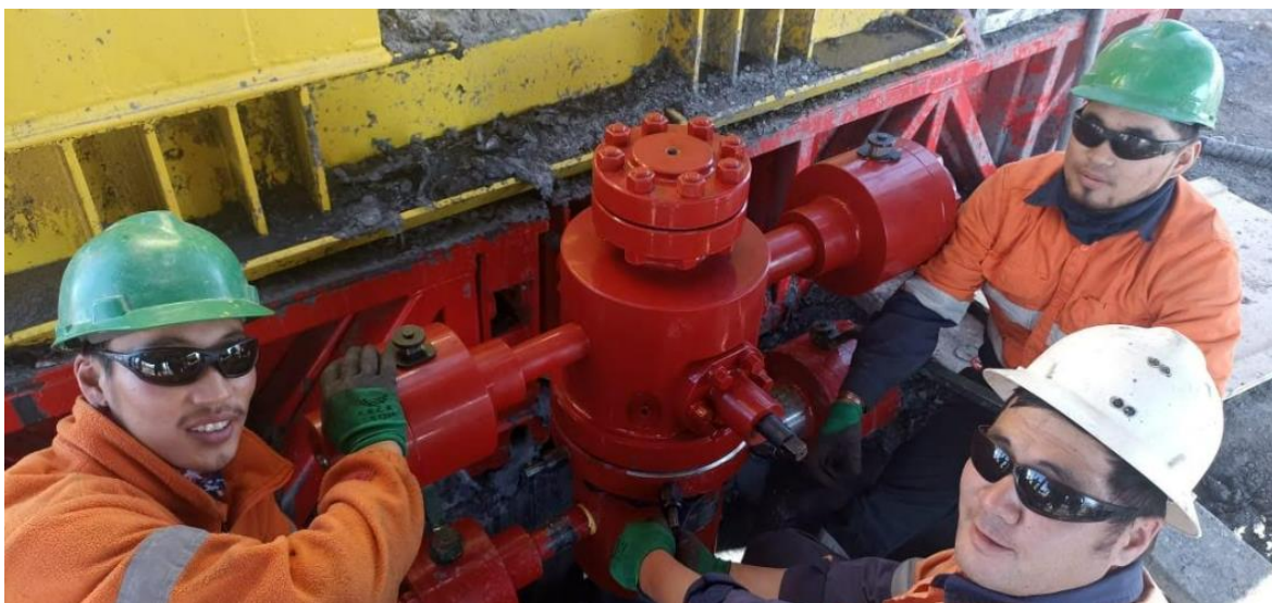
Wellhead installation at Nomgon-9
