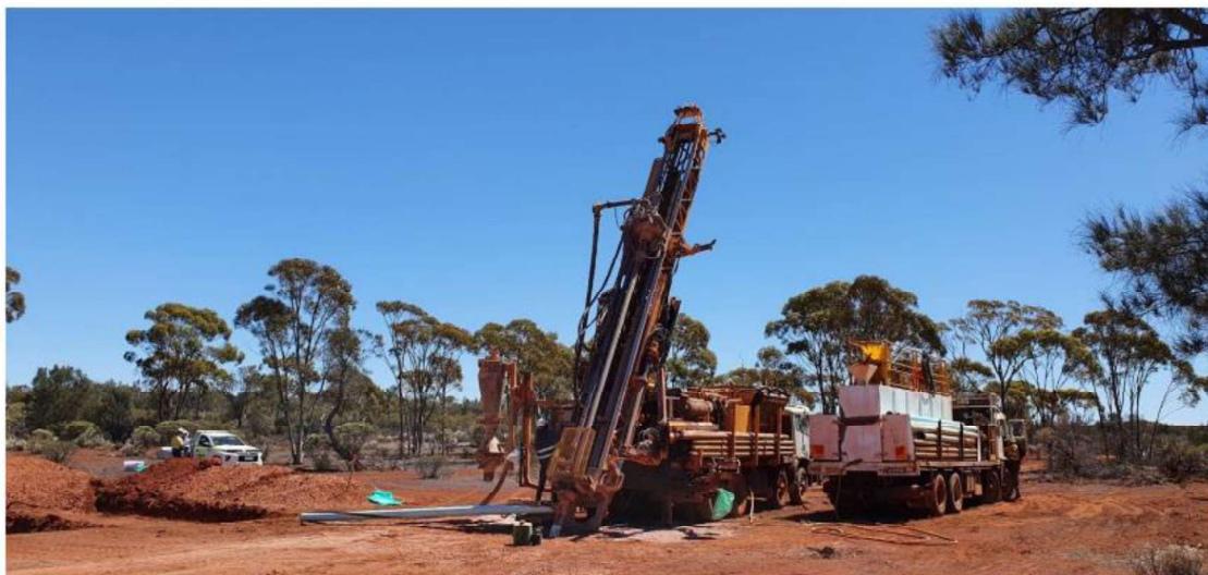
Figure 5: RC rig set up for drilling at Omrah nickel prospect
