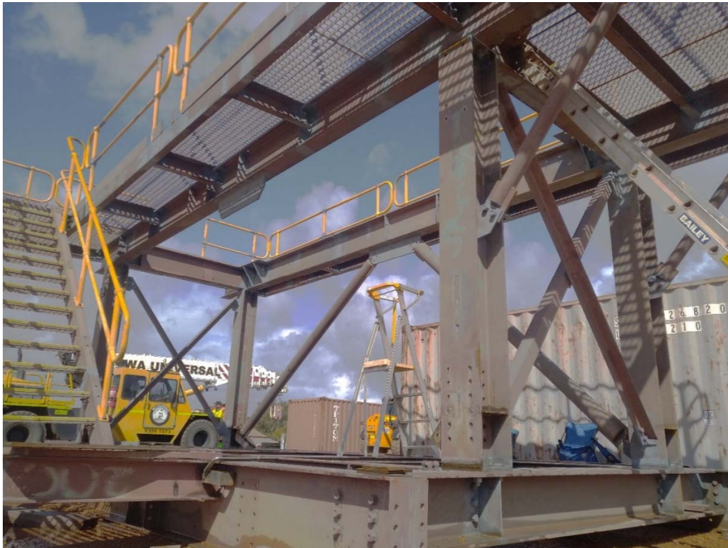
Steel Skid for the screw-press (to be inserted in centre of top level)
