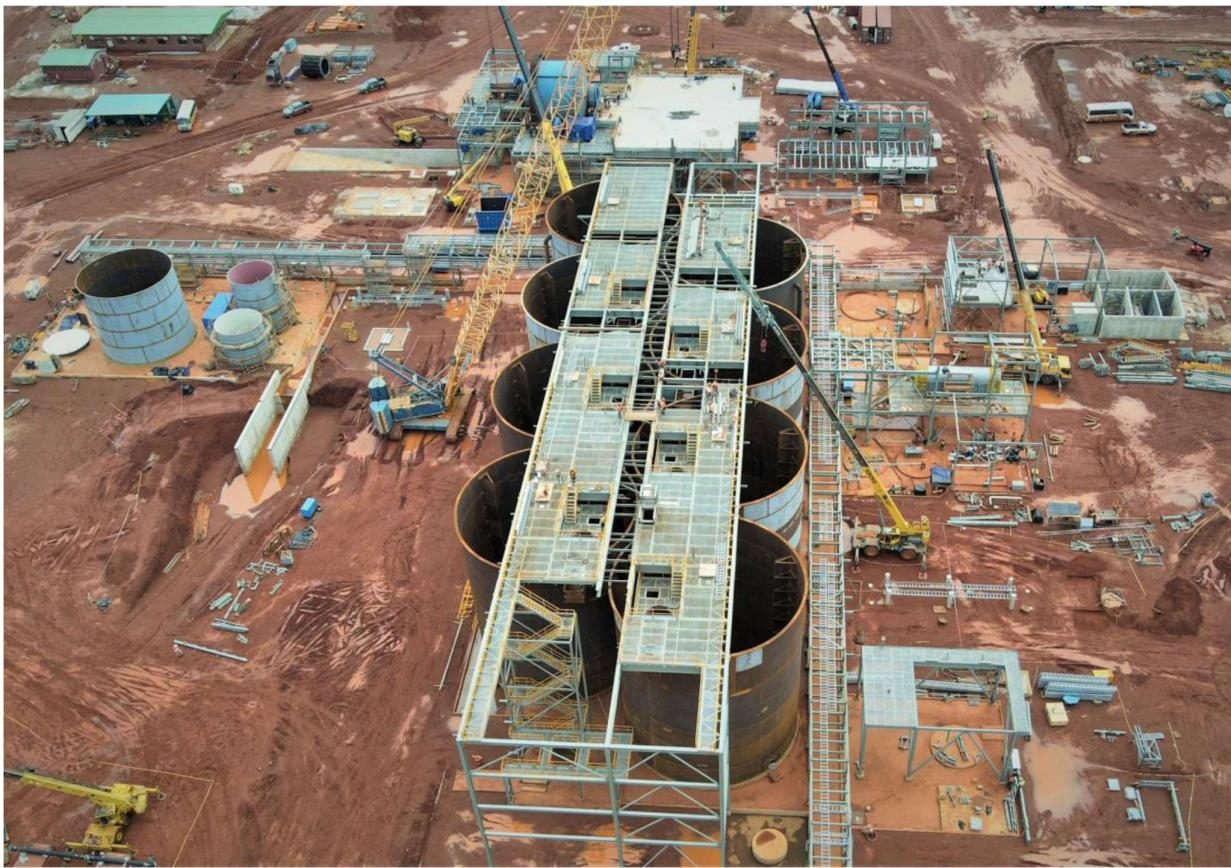
*Figure 4 CIL tanks installed*
