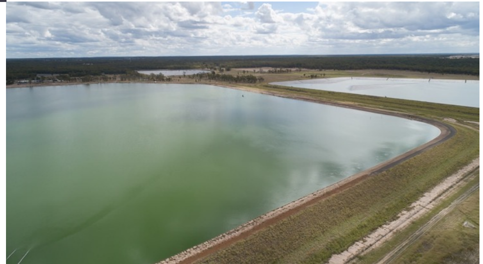
Waste brine ponds from gas production in Queensland, Australia.
