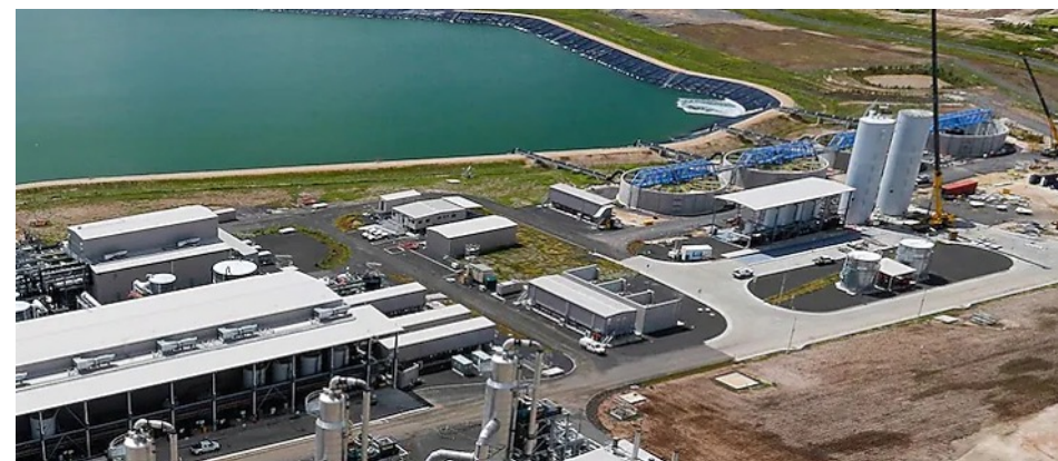
QGC Shell - Kenya Water Treatment Plant, in Queensland, Australia.
