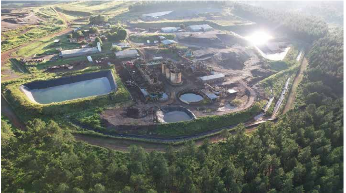
Figure 9: Existing Plant Drone View (post demolition of old sections)
