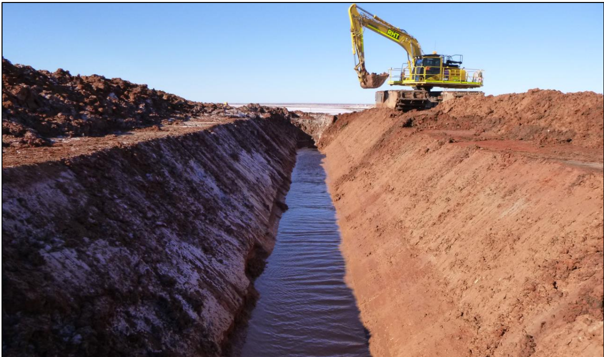
Figure 1. Trench Construction Trial in Progress
