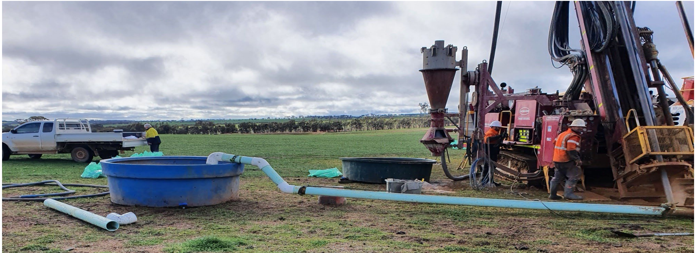
Example of an above ground sump to capture drilling water
