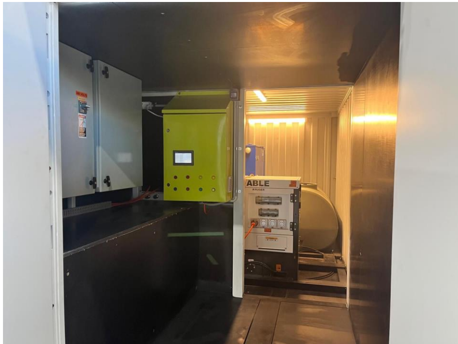
Figure 2: One of two production skids, showing the hydraulic power unit to drive the wellhead pumps for the pilot wells
