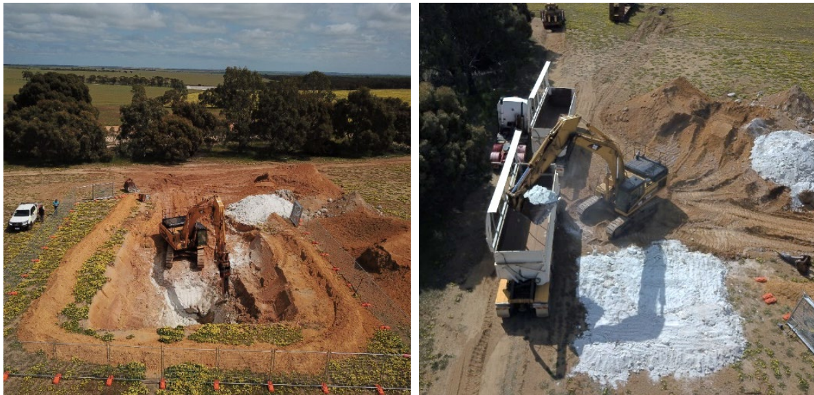
Figure 1: Test-pit in progress
